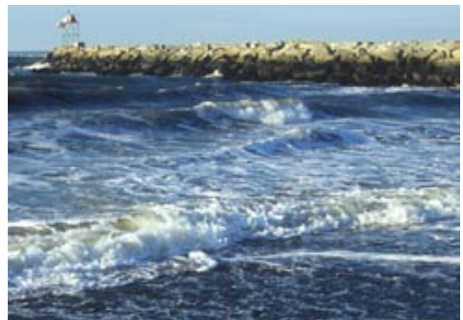
Jetties can cause erosion of beaches by disrupting the currents that transport and deposit sediments along the shore. Ethan Nedeau
