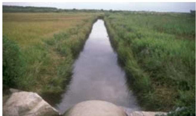
Tidal creek straightened to drain marsh and control mosquitoes. Ethan Nedean
